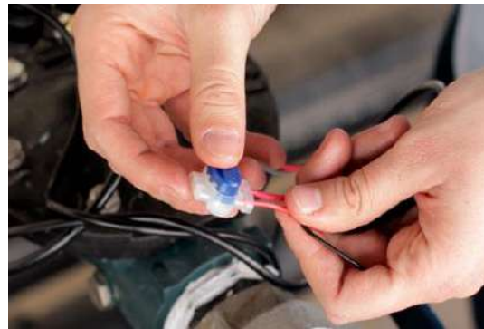
Figure 7 Connection of positive polarity by a sealed connector.
